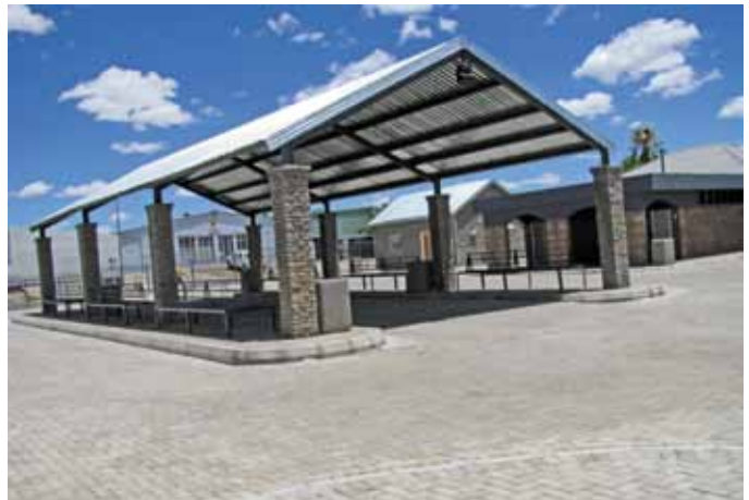
Completed Taxi Rank in De Aar
