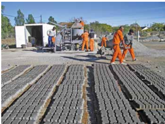
Manufacturing of pavers for streets
