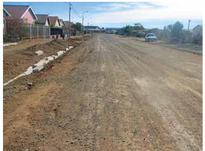
Kerbing and Channelling of Topaaslaan
