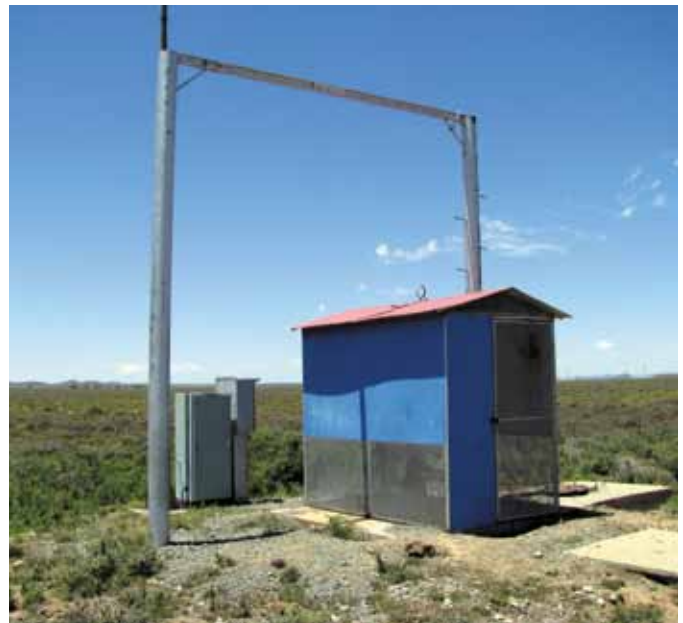
Well maintained borehole at Riet Water Scheme
