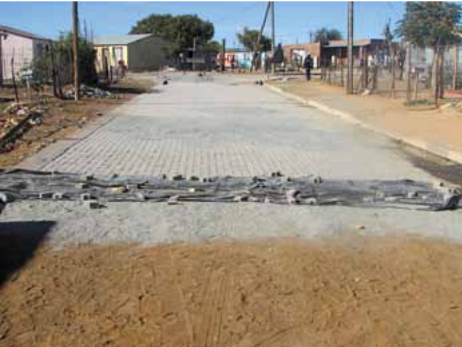
Paving and channelling of Street 8
