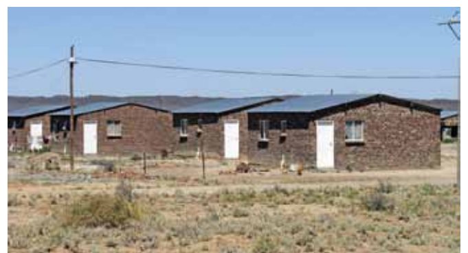
Britstown housing project
