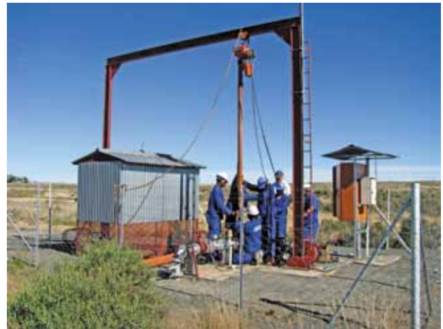
Waterworks Division staff busy with maintenance work on a borehole pump.
