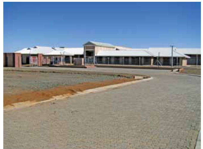
Newly Completed Secure Care Centre in De Aar
