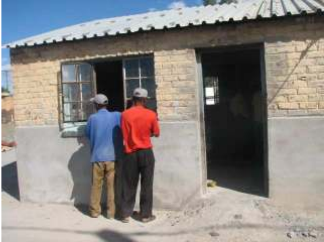
Workers busy with revitalization in Happy Valley
