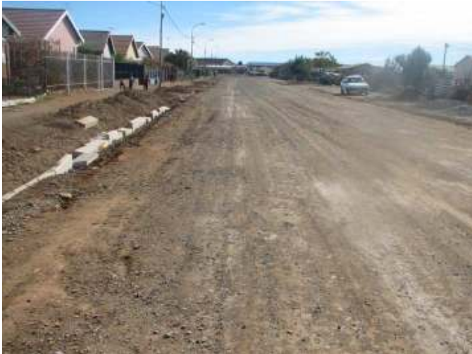
Kerbing and Channelling of Topaaslaan
