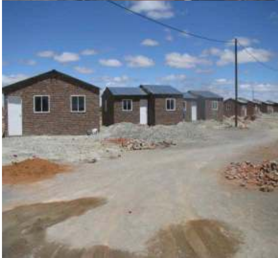
Hanover housing project – 100 houses 33 houses (Handing over of first houses)
