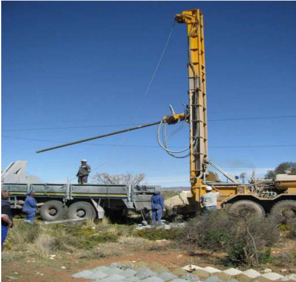
Drilling for new boreholes in Britstown
